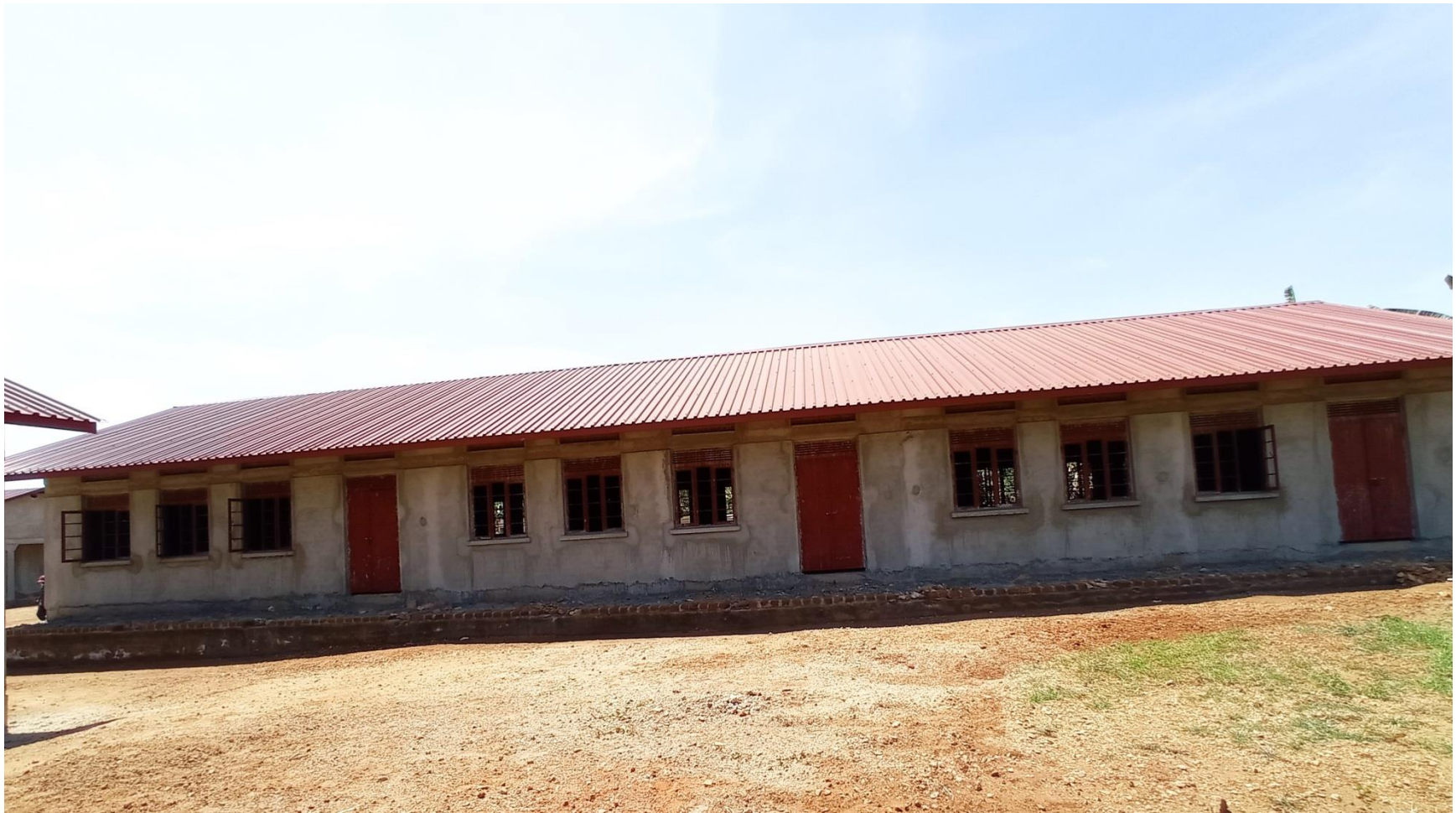
ONGOING CONSTRUCTION OF MULTIPURPOSE HALL
