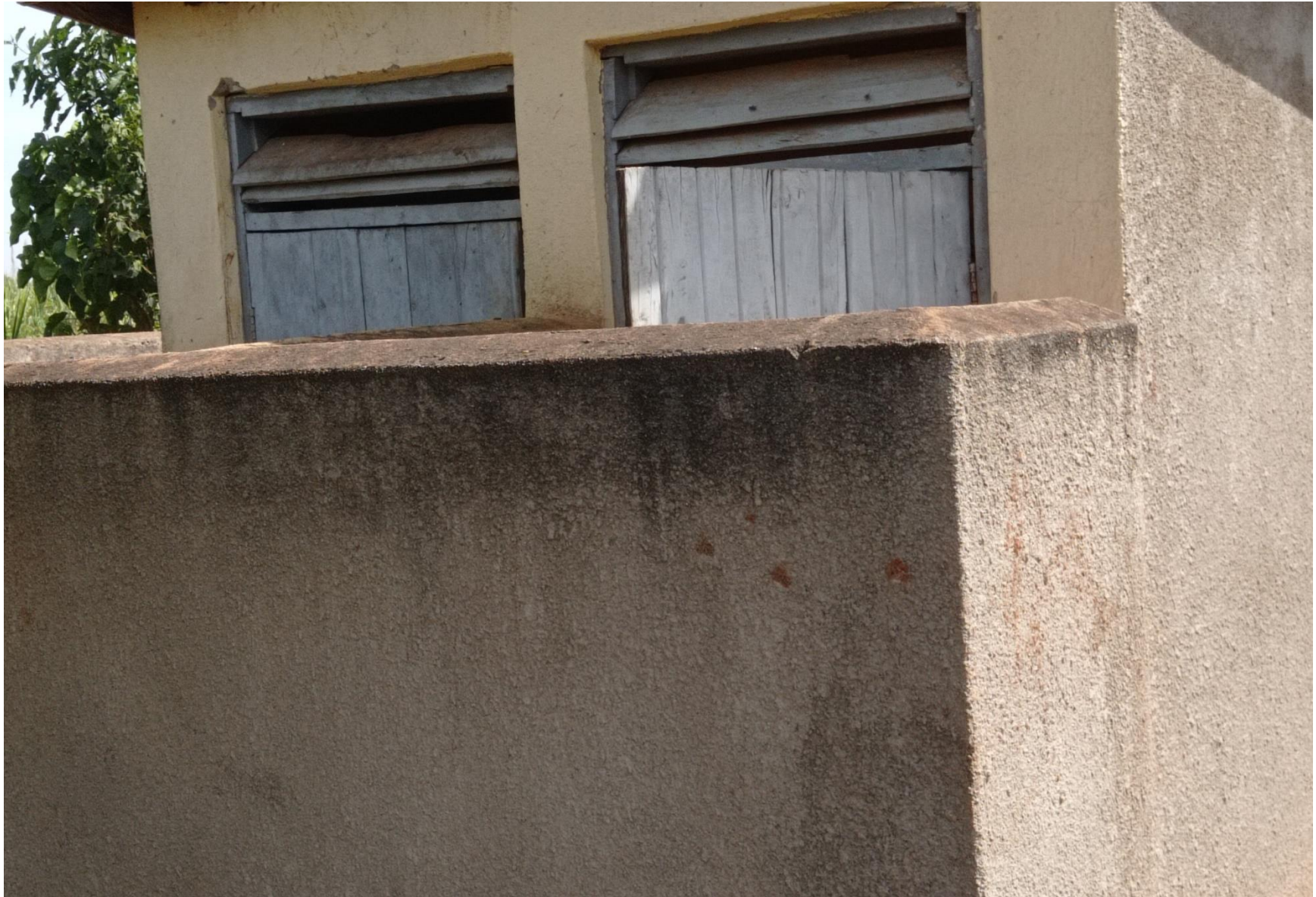
TWO STANCE PIT LATRINE AT NAMWENDWA SLAUGHTER SLAB
