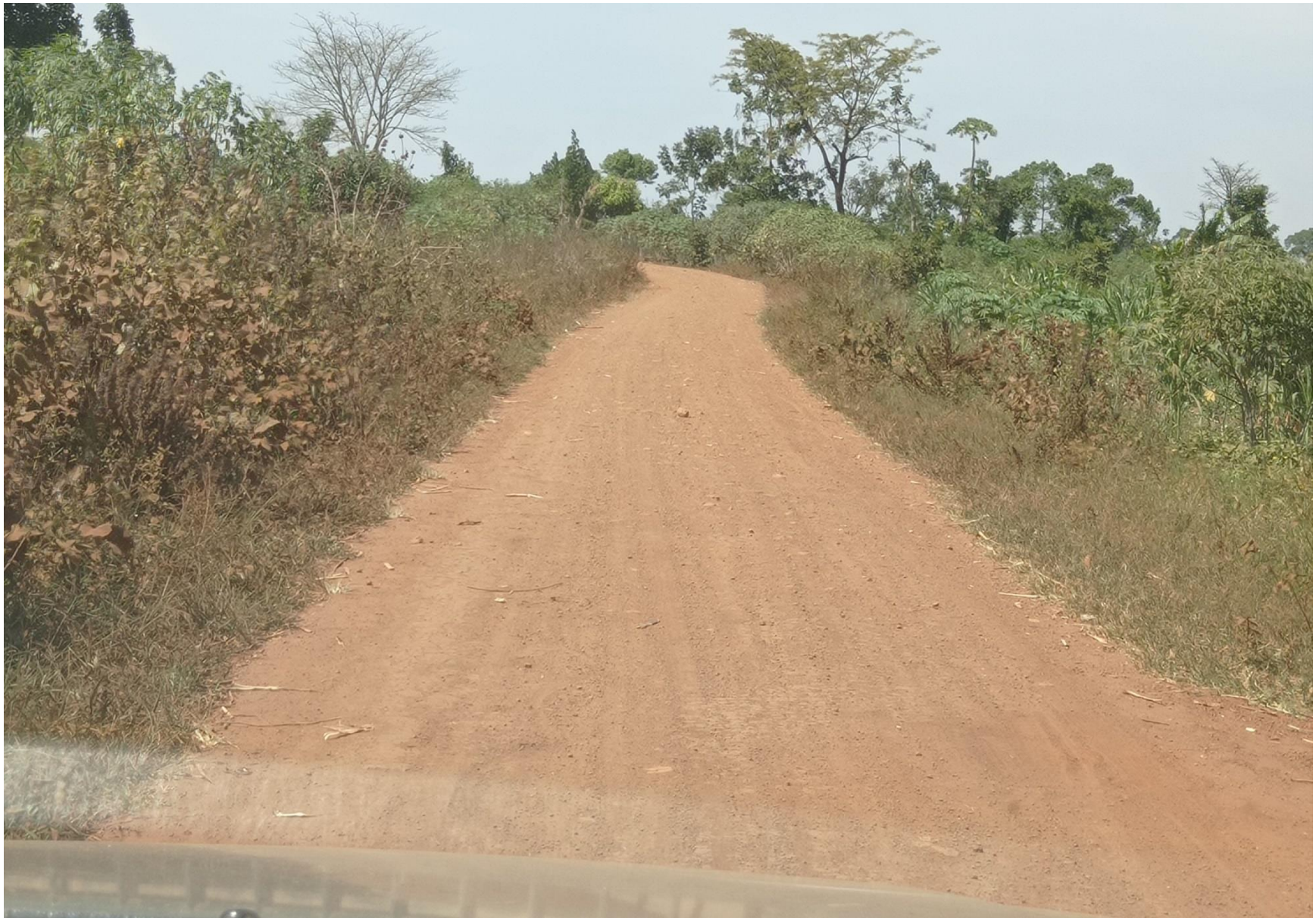
SECTION OF NABIRUMBA – BULOGO – BULOPA ROAD UNDER PERIODIC MAINTENANCE
