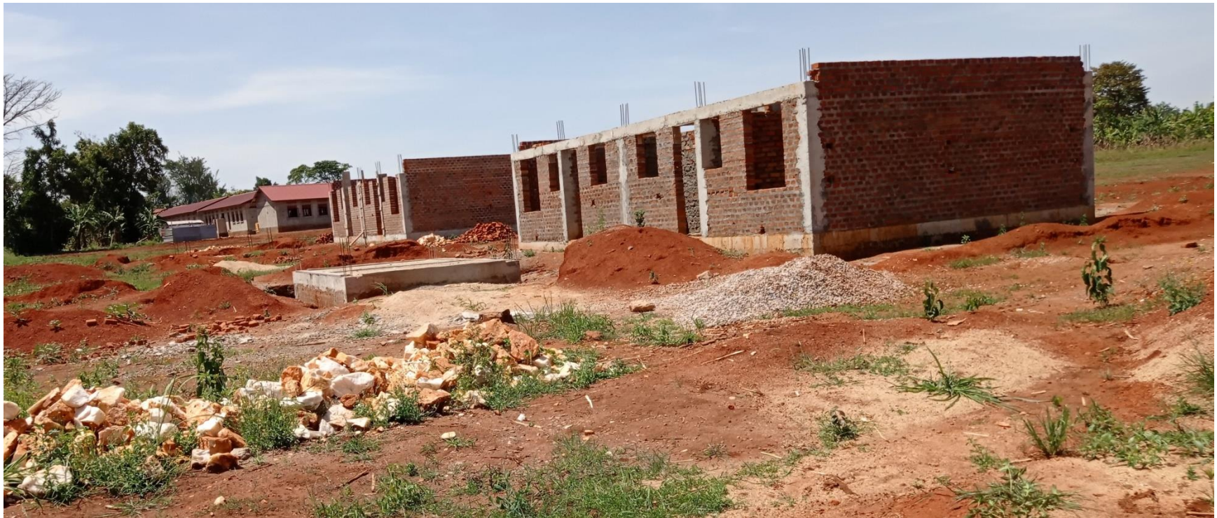
ONGOING CONSTRUCTION OF STAFF HOUSES (Blocks 1 & 2) - Back Elevation
