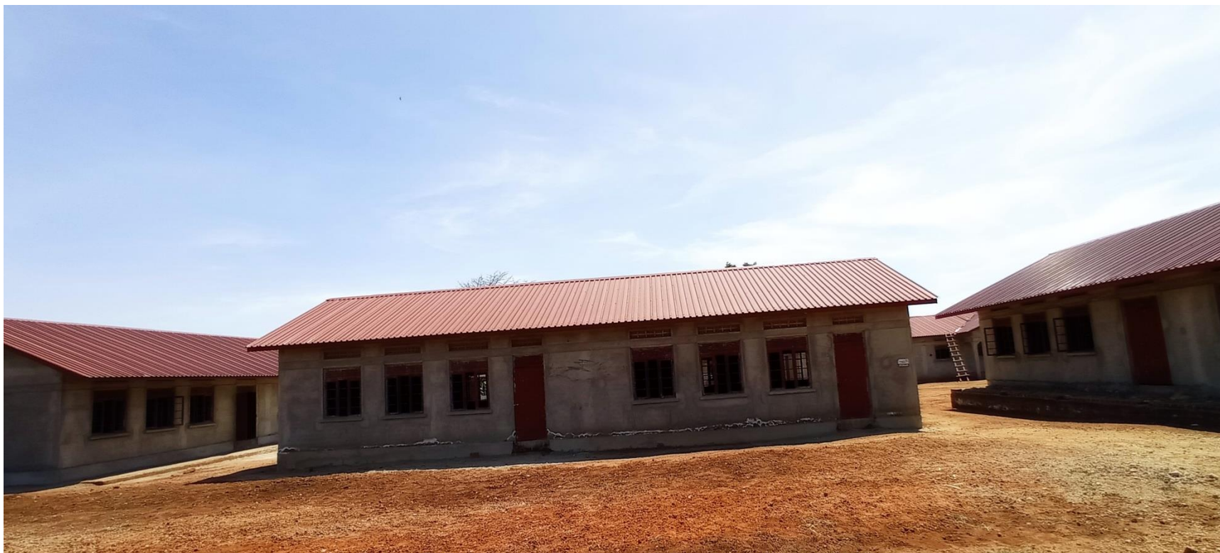
ONGOING CONSTRUCTION OF CLASSROOM BLOCKS
