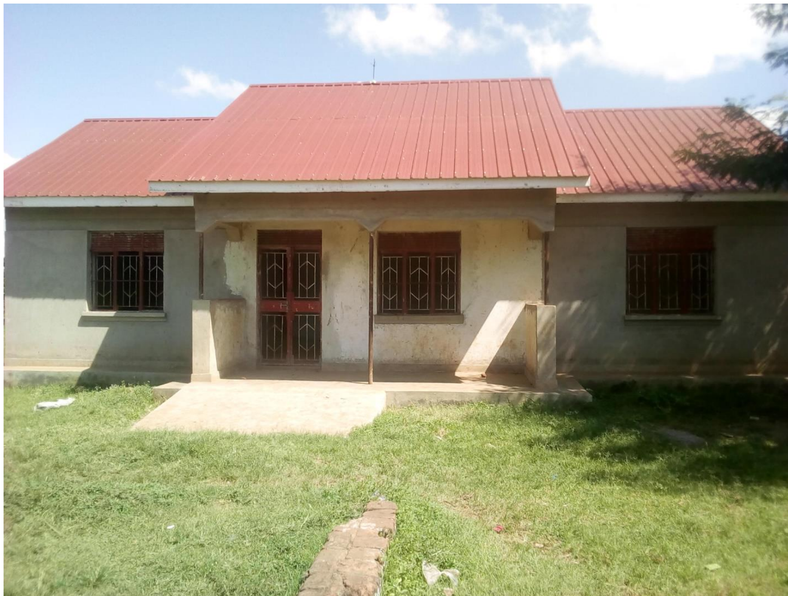
PARTIAL CONSTRUCTION OF MATERNITY WARD AT KASAMBIRA HC II, BUGULUMBYA SUB COUNTY
