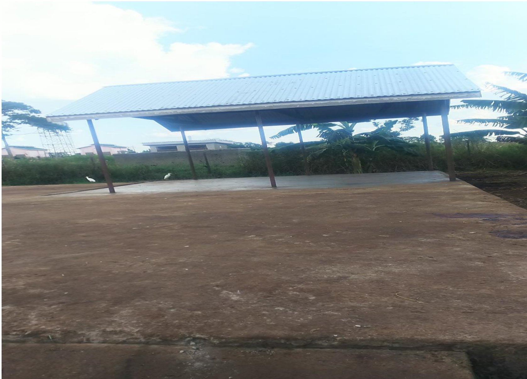
CONSTRUCTION OF A SLAUGHTER SLAB WITH TWO STANCE PIT LATRINE AND BATHROOM AT KISOZI SUB COUNTY
