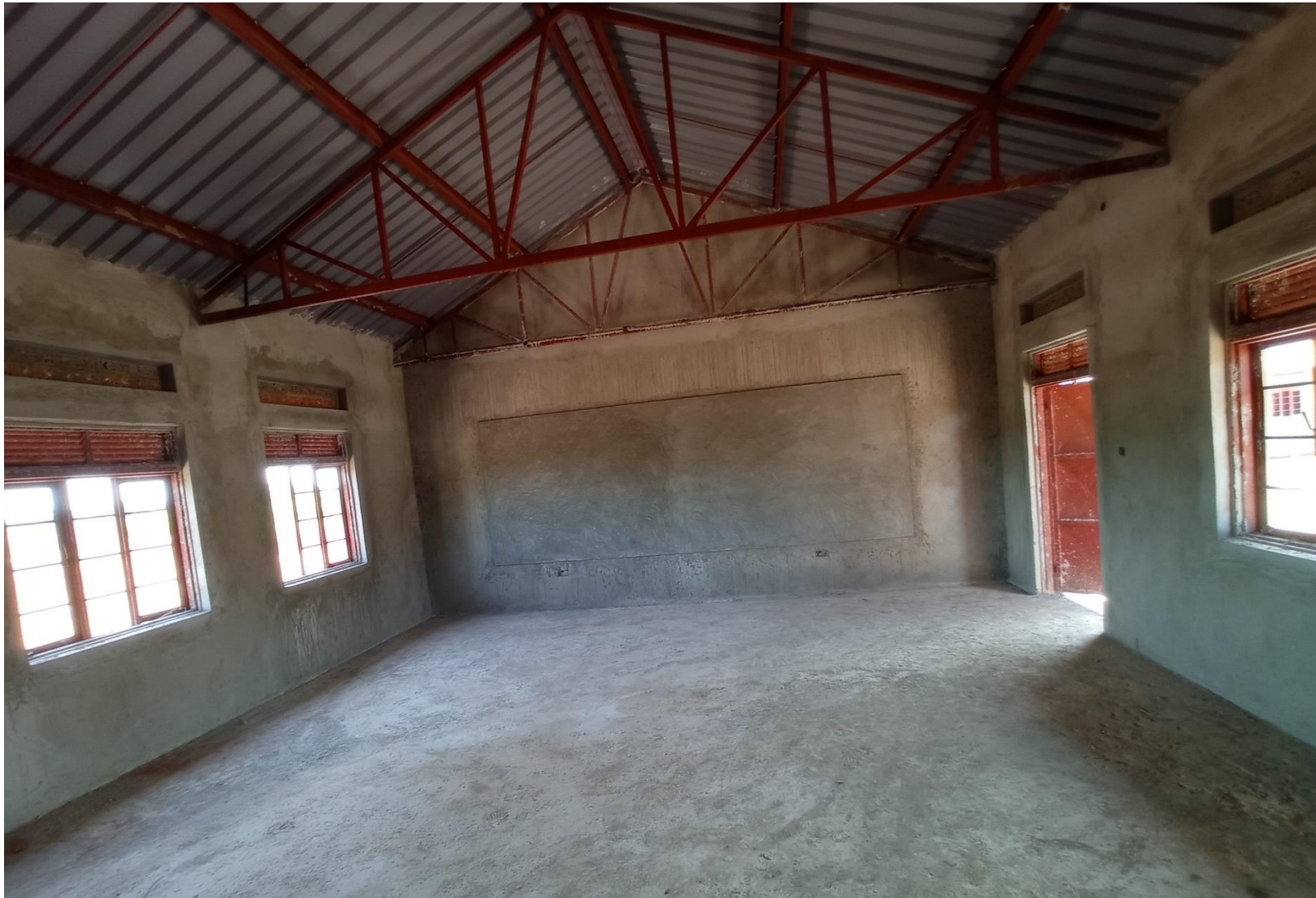
ONGOING CONSTRUCTION OF CLASSROM BLOCKS - INTERIOR
