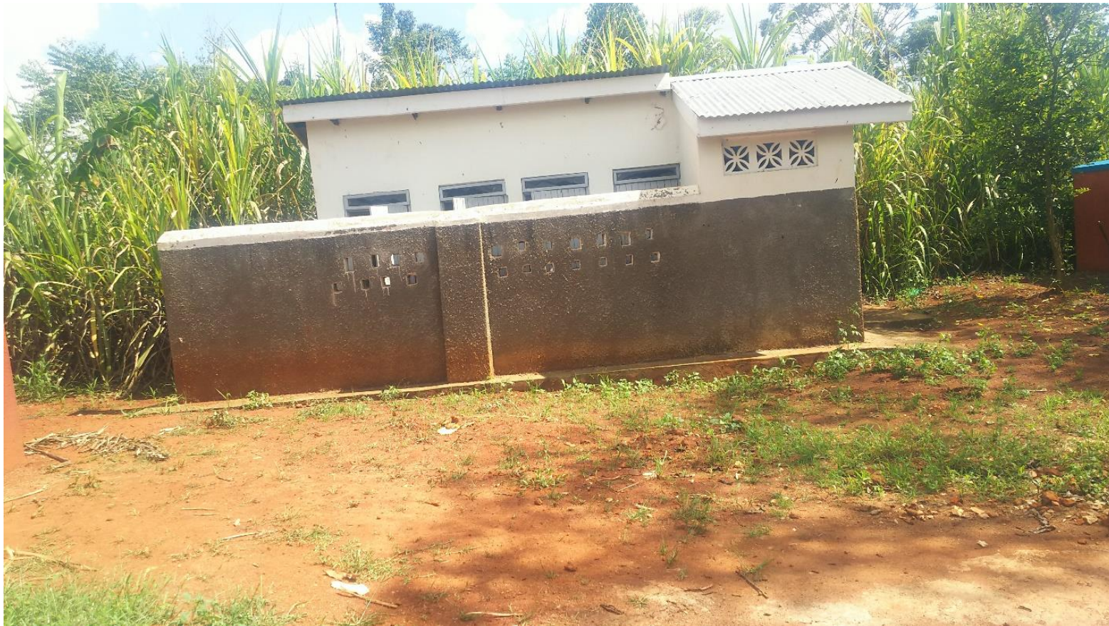
CONSTRUCTION OF A 5 – STANCE PIT LATRINE AT ITUKULU PRIMARY SCHOOL, NAWANYAGO SUB COUNTY
