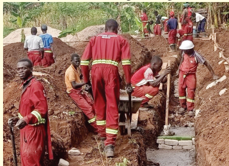
Contruccion work in progress
