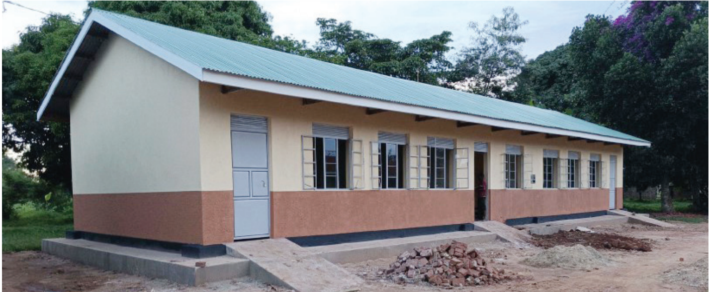
The picture above shows a newly constructed two classroom block with store and office at Bugulusi Primary School in Mbulamuti Sub County.
